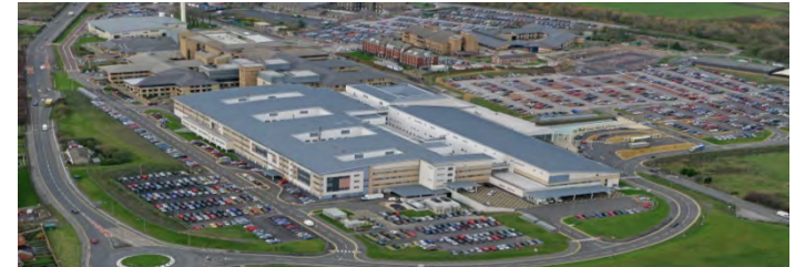
Blackburn Hospital - Emergency Dept extension
