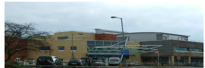
W Middlesex Hospital - A&E extension + M&E enhancements
