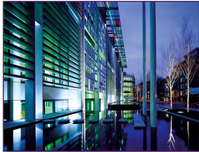
Home Office Headquarters
