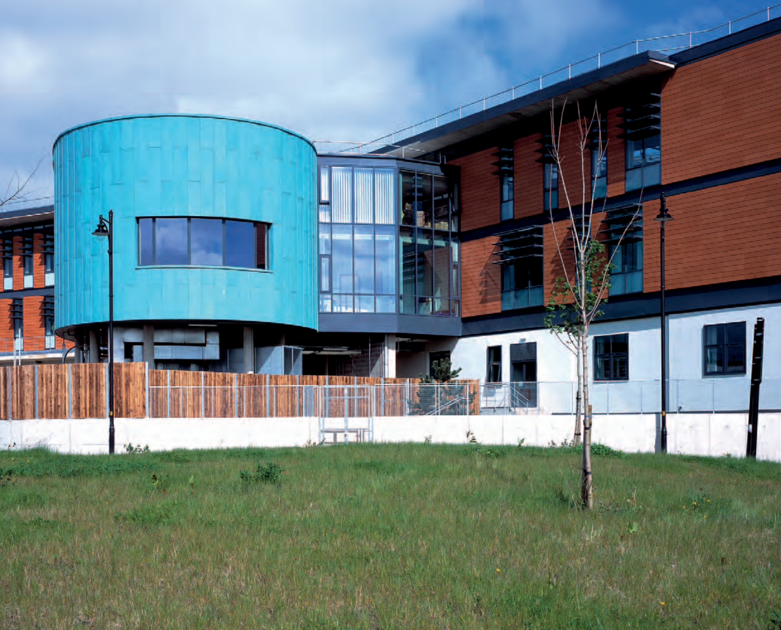
Oldham Library project, England
