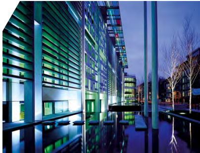
Home Office Headquarters
