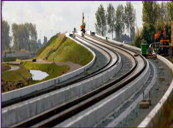
Dutch High Speed Rail Link, The Netherlands
