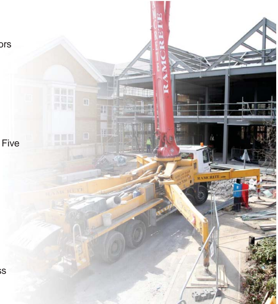
Picture – construction work at Barnet Hospital - variation
