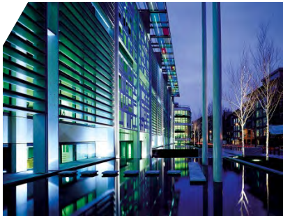
Home Office Headquarters
