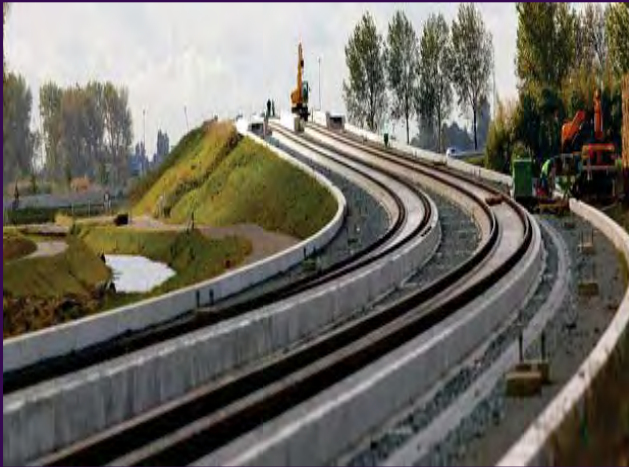
Dutch High Speed Rail Link, The Netherlands
